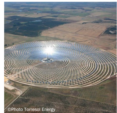
©Photo Torresol Energy
