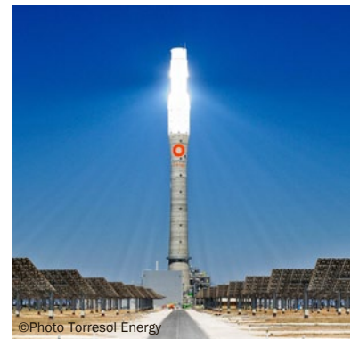
©Photo Torresol Energy
